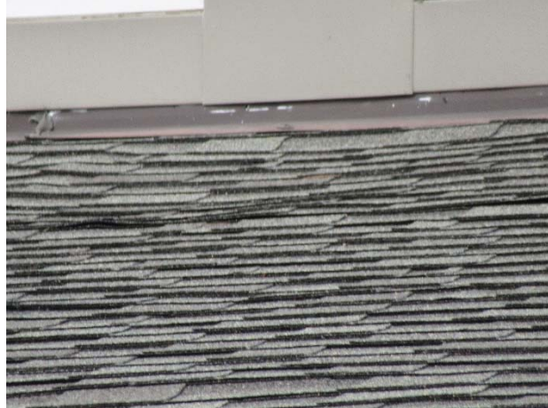
Shingle lift at Cardinal Lane
